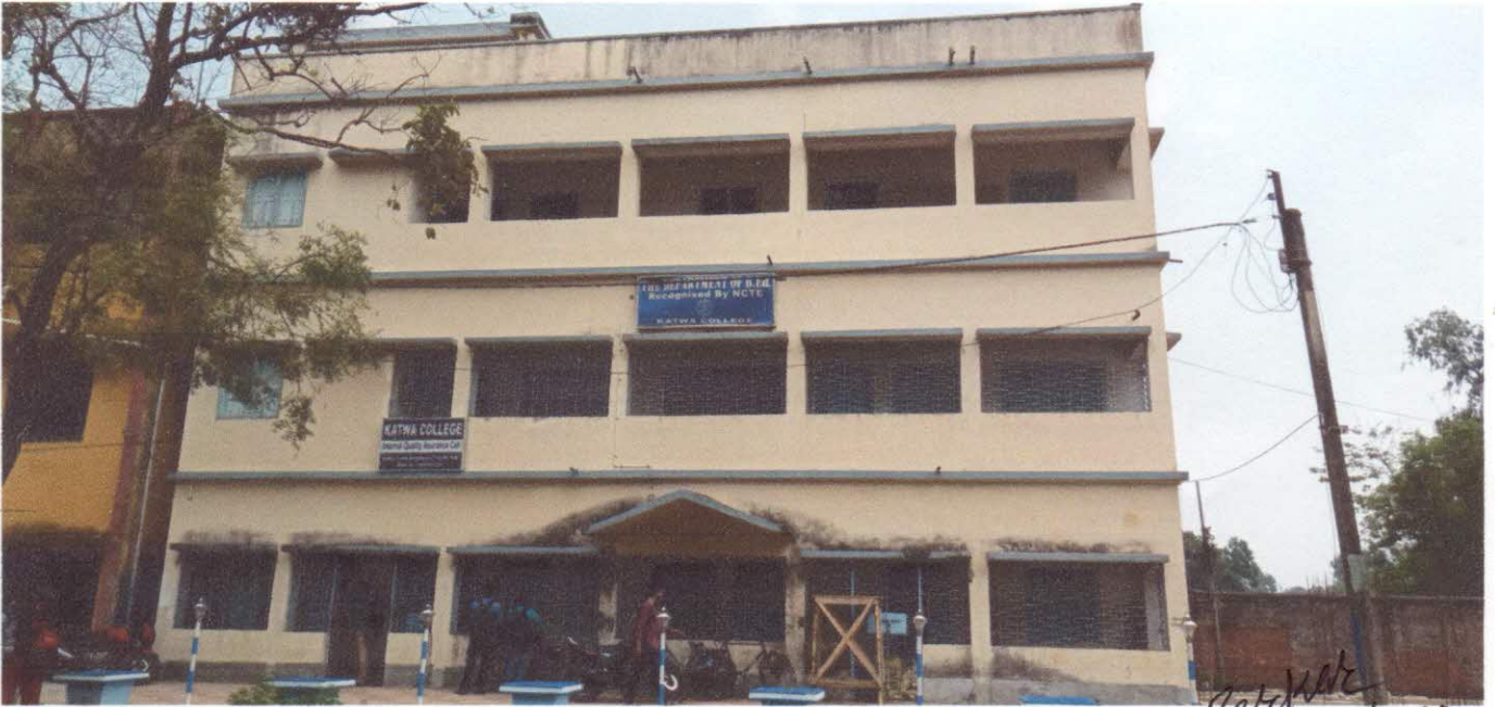
B.Ed Building Front
