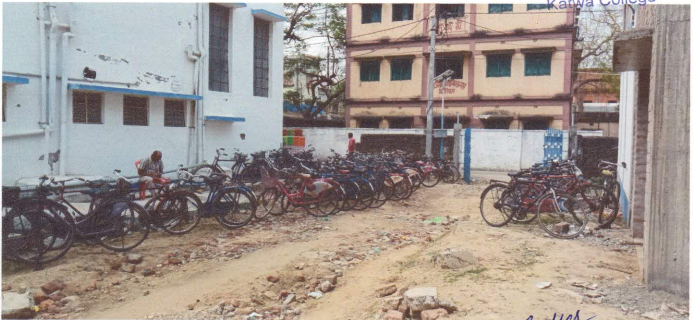
Parking (Under Construction)
